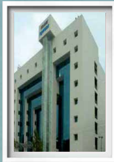
Trans Towers Vazhuthacaud, Tvm
