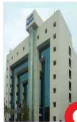
Trans Towers Vazhuthacaud, Tvm
