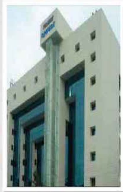
Trans Towers Vazhuthacaud, TVM
