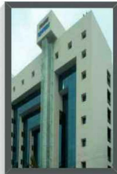
Trans Towers Vazhuthacaud, TVM
