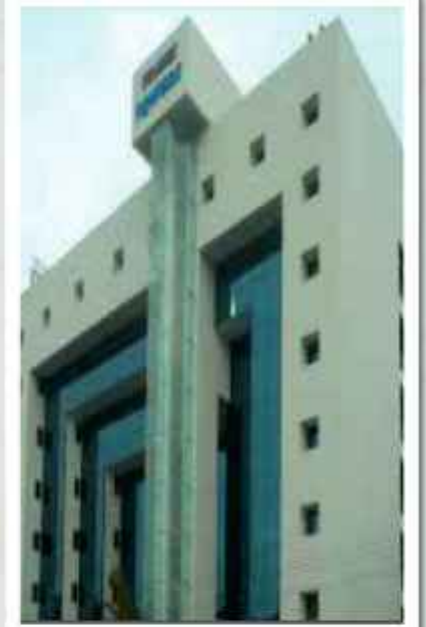
Trans Towers Vazhuthacaud, TVM
